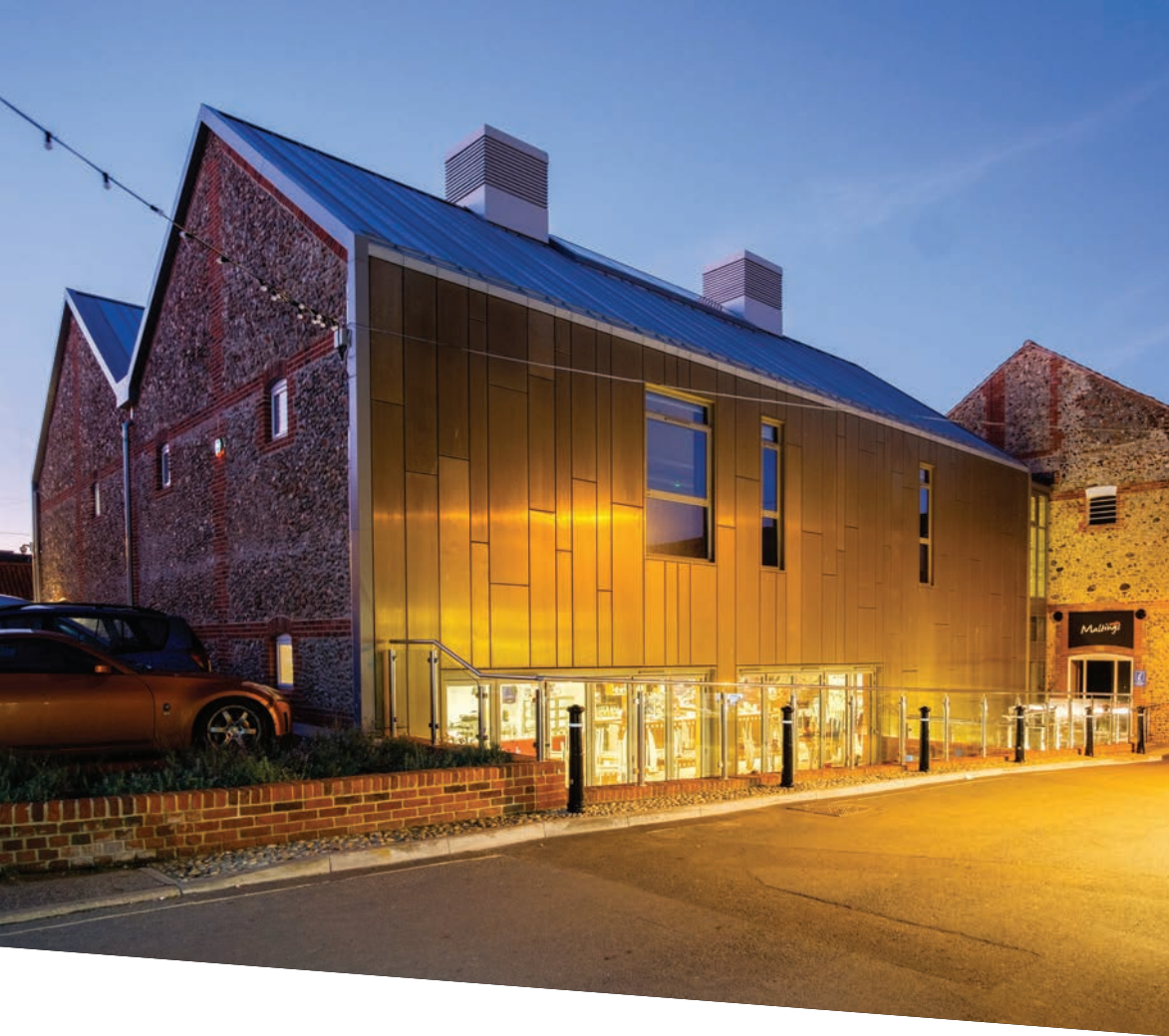
OPPOSITE : Robson Construction's award-winning Holkham Lookout at the end of Lady Anne's Drive on the Holkham Estate.
